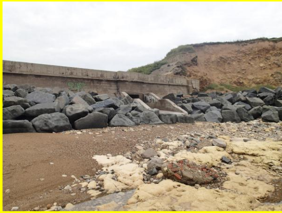
Culverted outfall from Dawdon Dene. (Asset Ref. No. 121AC901C0103C04)
