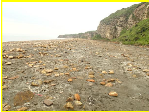
Eroding spoil at north end of Blast beach. (Asset Ref. No. 121AC901C0107C01)
