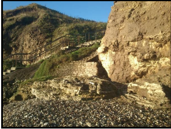
Photo from 2012 report. (Asset ref. No. 121AB901B0804C01)
