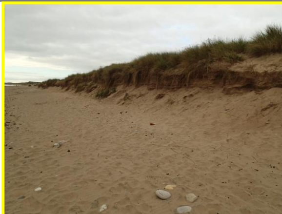
Evidence of erosion of front face of dunes. (Asset Ref. No. 121AC901C0301C02)
