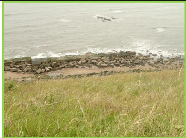
Rock armour bund seaward of cliff. (Asset Ref. No. 121AC901C0105C01)
