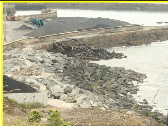
Rock armour at root of South Pier. (Asset Ref. No. 121AC901C0104C01)
