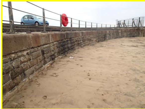
Low masonry wall at back of beach. (Asset Ref. No. 121AC901C0104C05)
