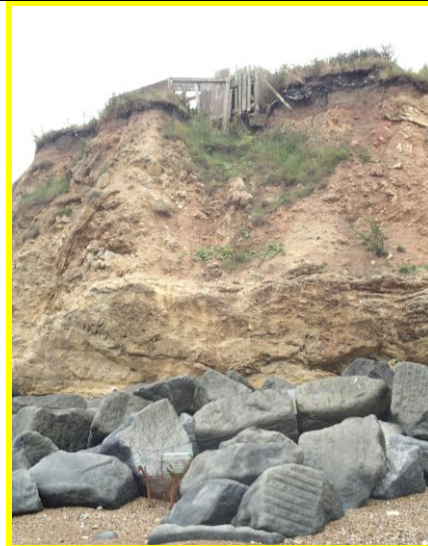
Ongoing erosion of cliff behind rock armour. (Asset Ref. No. 121AC901C0103C02)
