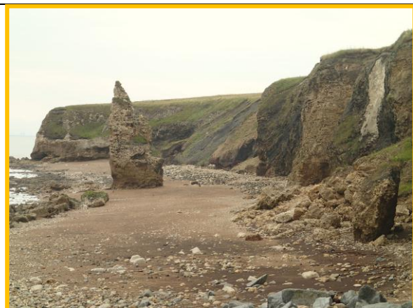
Colliery spoil has been eroded from Chemical Beach. (Asset Ref. No. 121AC901C0106C01)
