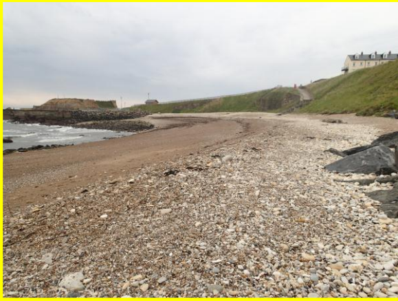
Beach remains high at cliff toe but has steepened since 2012. (Asset Ref. No. 121AC901C0103C06)
